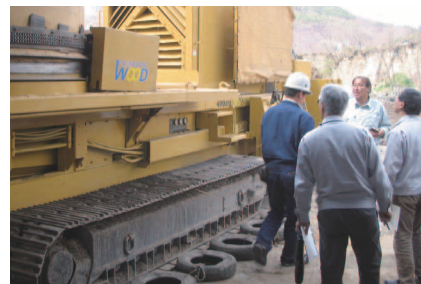
The situation of on-site inspection
