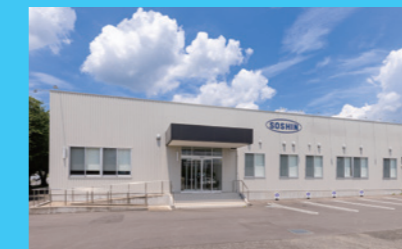
5 Miyakonojo Plant (formerly known as Soshin Powertech)
