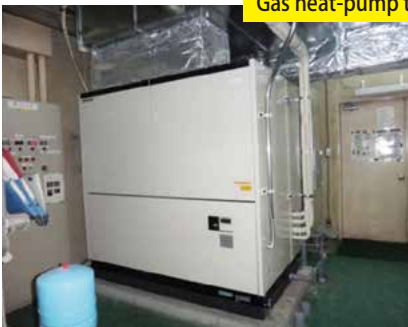
Gas heat-pump type air conditioner
