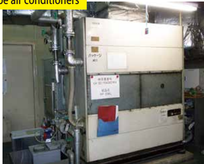
Electric package type air conditioners
