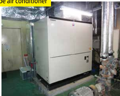
Gas heat-pump type air conditioner
